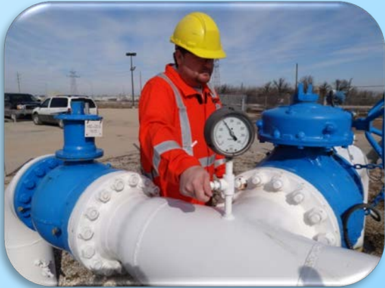
Natural Gas Equipment inspections
