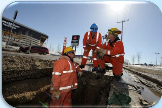
Natural Gas Maintenance & repairs
