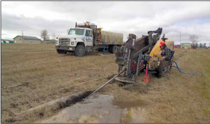
Directional boring new services.
