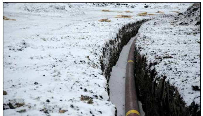
Installation of new natural gas transmission lines.
